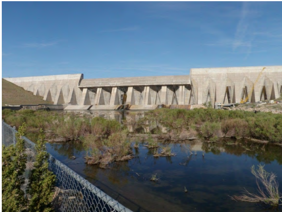
Figure 2 - Downstream view of Pueblo Dam and spillway.
