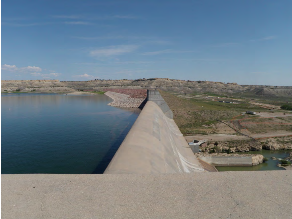
Figure 3 - Pueblo Dam uncontrolled spillway in center portion of dam's concrete section.
